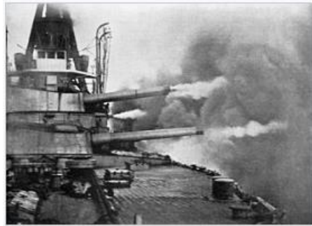
The gun trials of the Brazilian dreadnought Minas Geraes in 1910, where all the guns capable of training to the port side were fired, forming what was at that time the heaviest broadside ever fired from a warship
